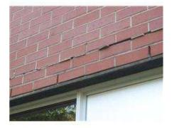
August 2012 - Missing mortar joint of exterior wall noted
