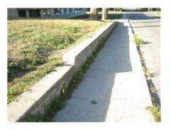
August 2012 - Cracked concrete paved walkway noted
