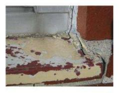
August 2012 - Deteriorated window perimeter sealant noted
