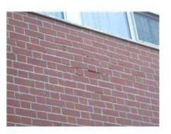
August 2012 - Deteriorated mortar joints noted
