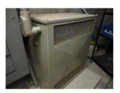
2012 - The transformer has exceeded expected useful life. Failure of the transformer can affect operation of the building. Replacement of the transformer is recommended.
